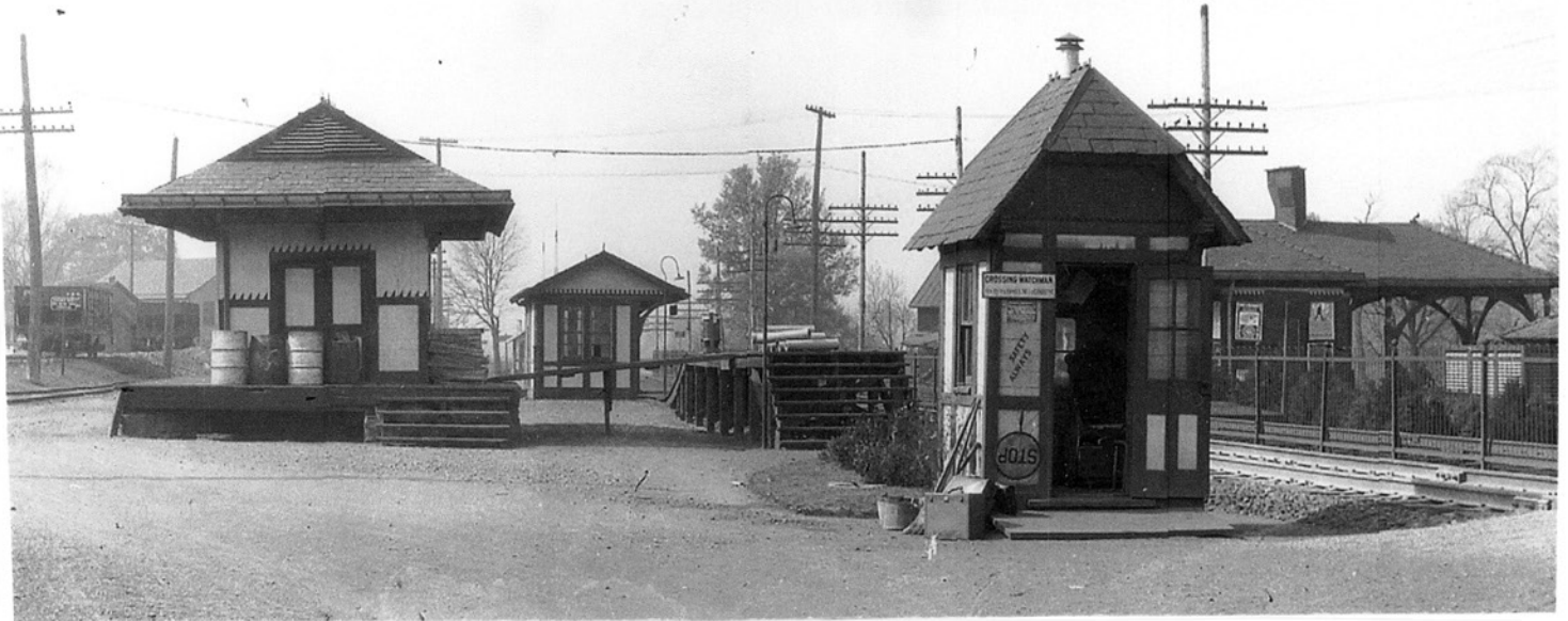
TOP PHOTO: A view of the Bethayres station area, undated, but prior to 1931, when electrification was installed as far as West Trenton, NJ. Today, only the station building (right rear) remains. Left to right: Freight house, outbound platform shelter, watchman shanty for Welsh Road crossing. Original photo by BRUCE G. SAYLOR, Collection of Larry Eastwood.
